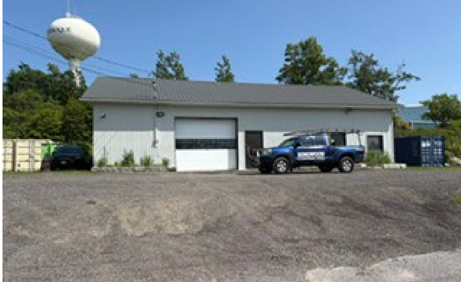
View of the Front of 215 James A. Brennan Road
